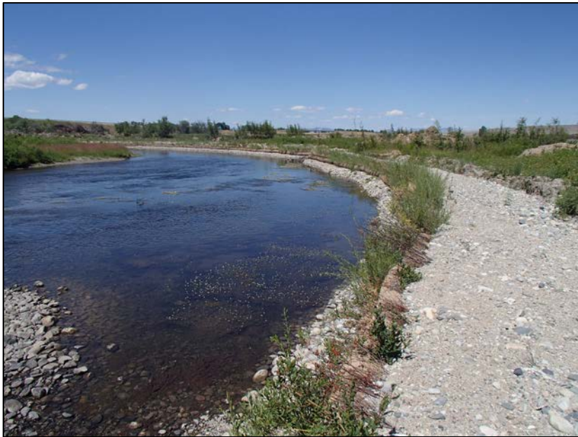
SUBSTRATE THAT ENCOURAGES WILLOW EXPANSION PLACED 10' BEHIND TREATMENT
